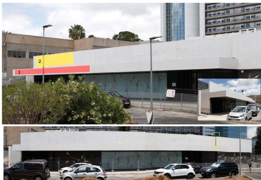
View of the ITB building in the first phase of construction on the Health Sciences Campus, located next to the School of Medicine and the University Hospital of the Canary Islands.
